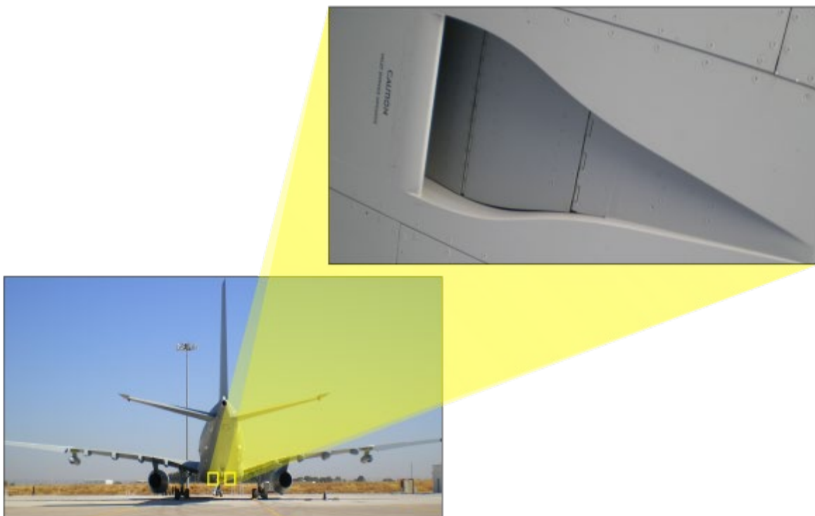
Figure 62 Outlets and inlets of the air conditioning system
